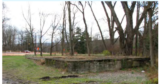
Fig. 2-79 Train Station platform — foundation remains and can be adapted to support a new multi-use pavilion The intersection of Bushkill Falls Road with US Route 209 is seen beyond.
