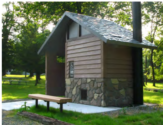
Fig. 2-129 The standard DEWA rest facility is a precast concrete waterless toilet that requires regular pumping. Bushkill Village has three of these units.
