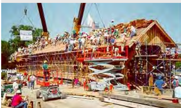
Fig. 3-19 The Timber Framers Guild convened to build the 120-foot Gift Covered Bridge in Ontario for the City of Guelph in 1992 .
